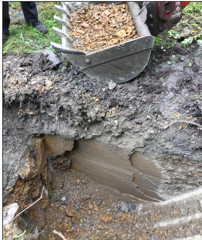
Plate 8: General view of TP5, and arisings of weathered rock in excavator bucket.
